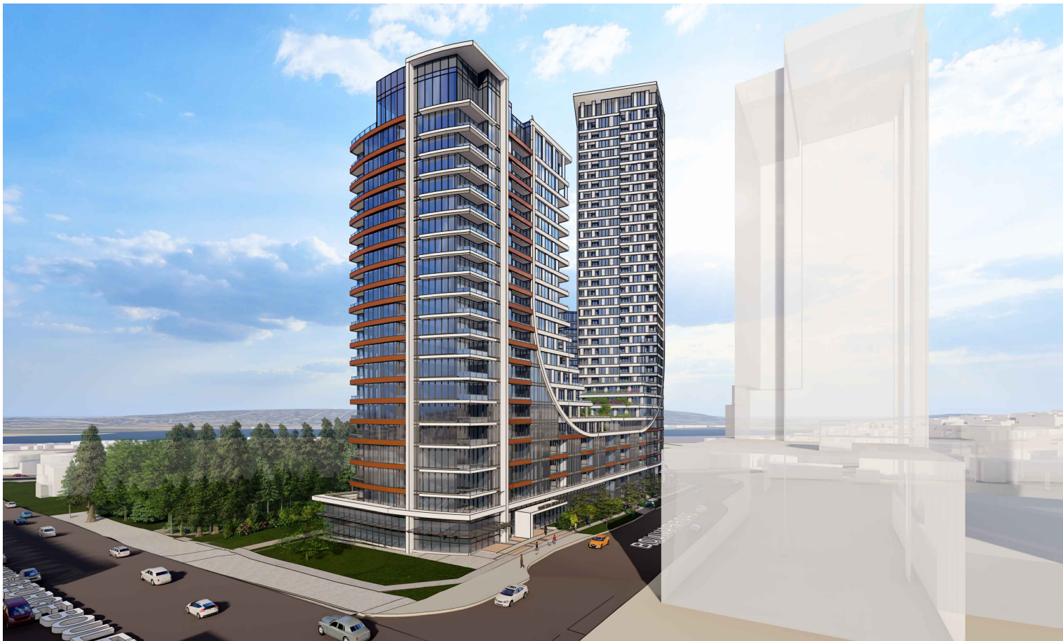
VIEW FACING NORTH WEST FROM THE CORNER JUNCTION AT KING GEORGE BLVD. AND BOLIVAR RD.
