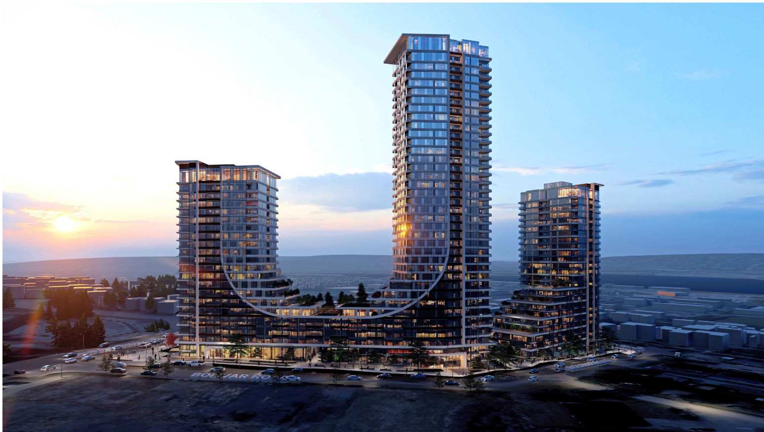
VIEW FACING SOUTH WEST FROM BOLIVAR ROAD
