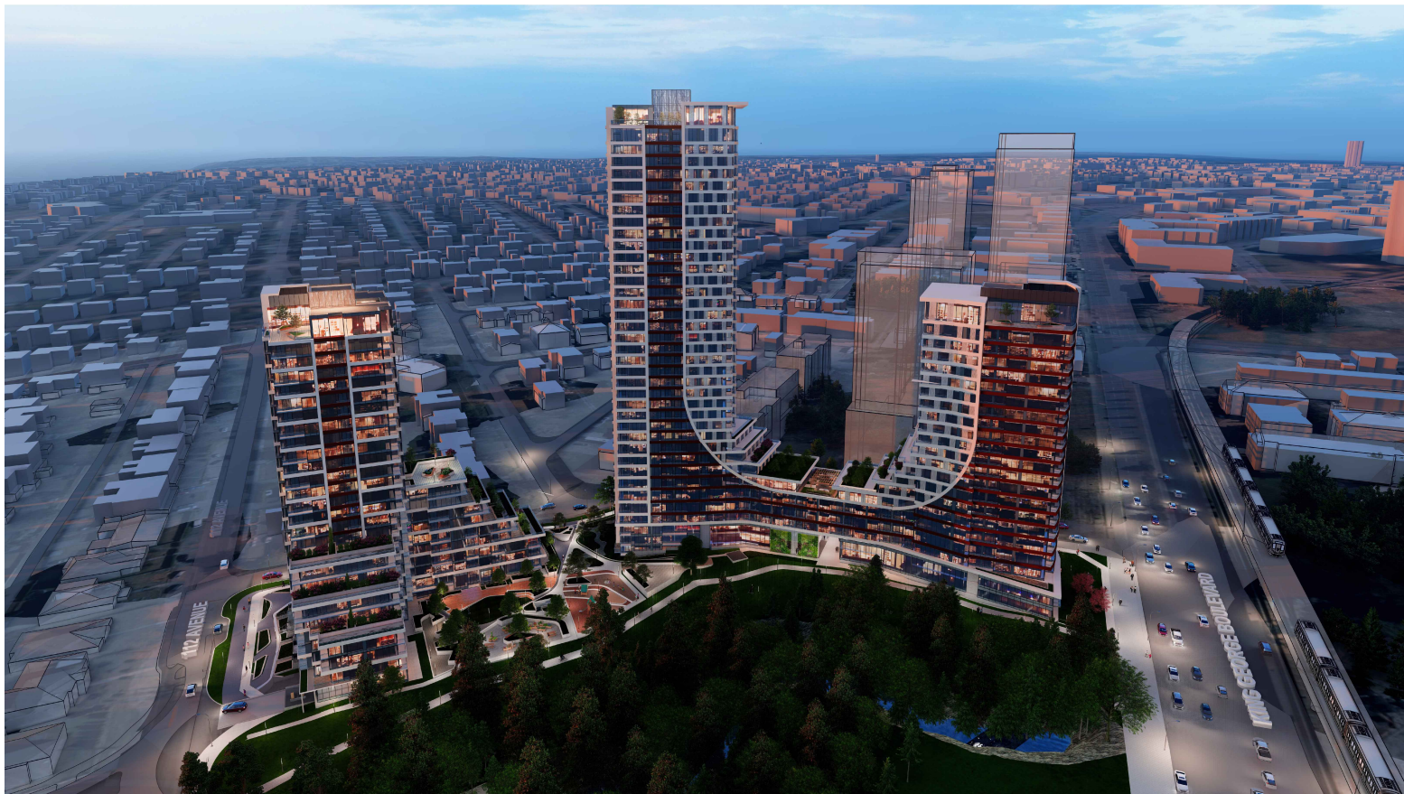
VIEW FACING EAST FROM BOLIVAR CREEK
