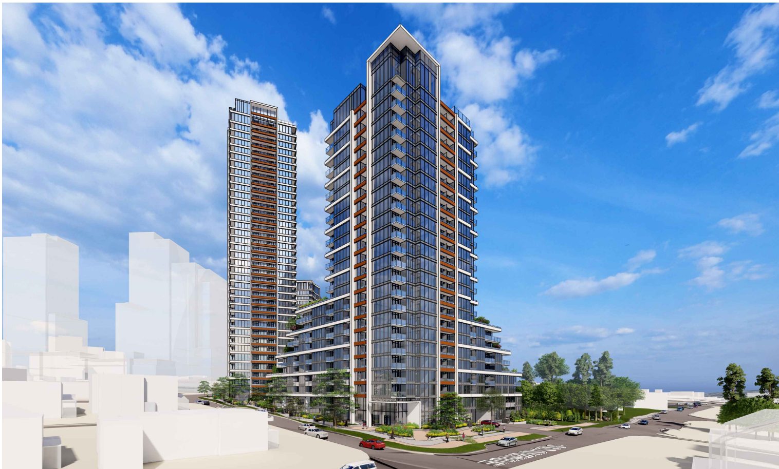
VIEW FACING SOUTH WEST FROM THE CORNER JUNCTION OF BOLIVAR ROAD AND 112 AVE.
