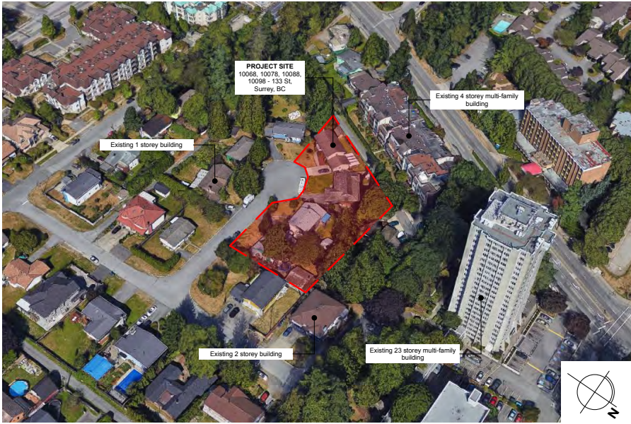
VIEW LOOKING FROM SOUTH-EAST
