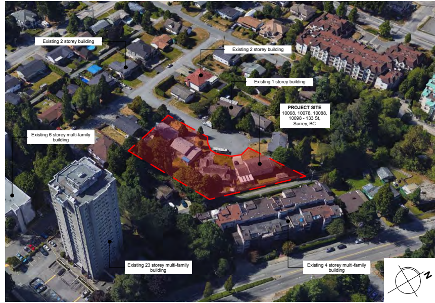
VIEW LOOKING FROM NORTH-EAST
