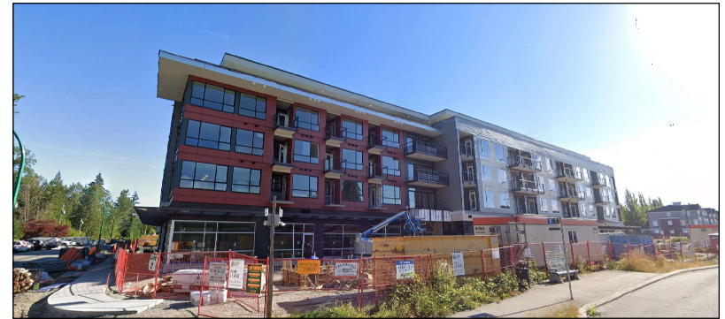
A 5 STOREY BUILDING @ 188 ST. AND 72 AVE.
