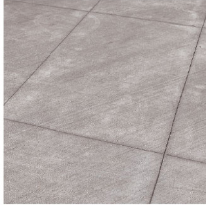
2 - SAW CUT CONCRETE NATURAL COLOUR, BROOM FINISH
