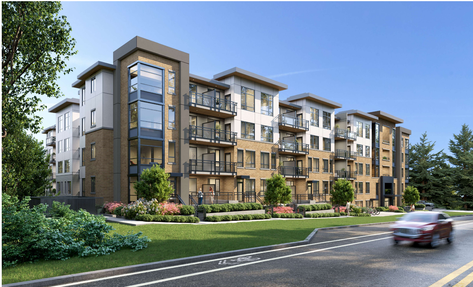
VIEW FROM NORTH-WEST CORNER
