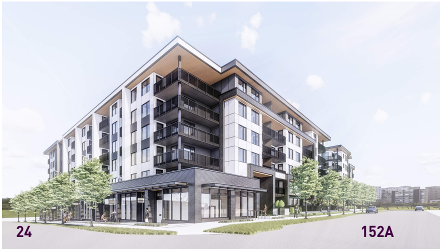
1: NORTH WEST CORNER
