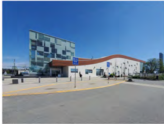
View from 107a Ave looking South East at the Existing Chuck Bailey Recreation Center main entrance
