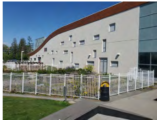
View of west facade from south, with view of community gardens
