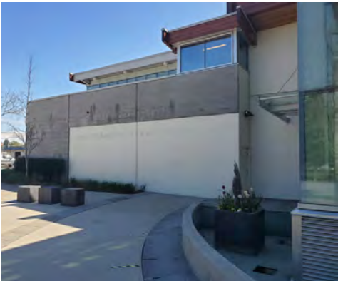
View of east main entry from 107A Avenue
