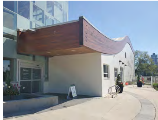
View of west facing main entry
