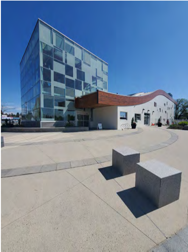
View of west main entrance from plaza at 107A Avenue
