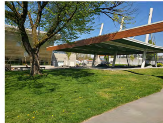
View looking North East at the skatepark, covered skate park canopy and the Existing Chuck Bailey Recreation Centre
