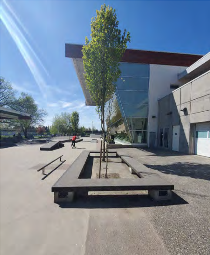
View of sloped gymnasium glazing from east
