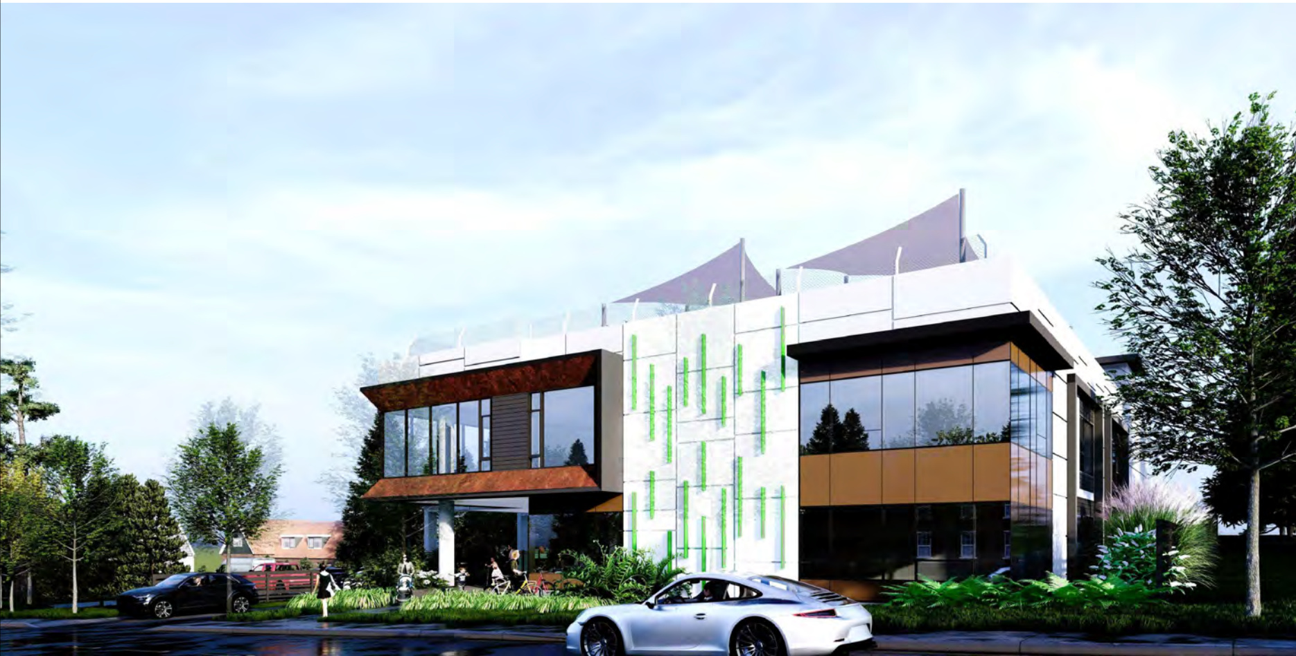
NORTH WEST CORNER VIEW
