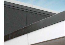
2. PREFIN. METAL FLASHING
