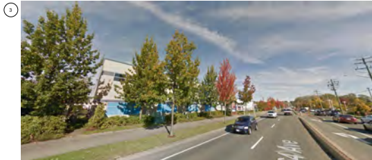
LOOKING NORTH - EAST FROM 64 AVENUE
