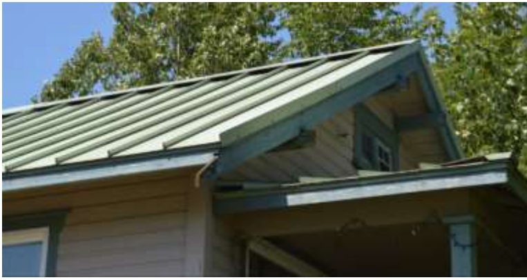
Figure 17: Standing seam metal roof
