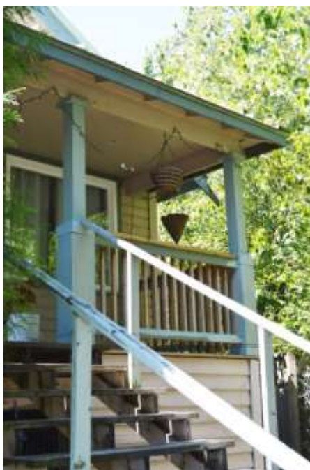
Figure 27: Porch posts, stairs and balustrade
