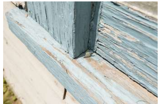
Figure 63: W09 Rail, Jamb and sill
