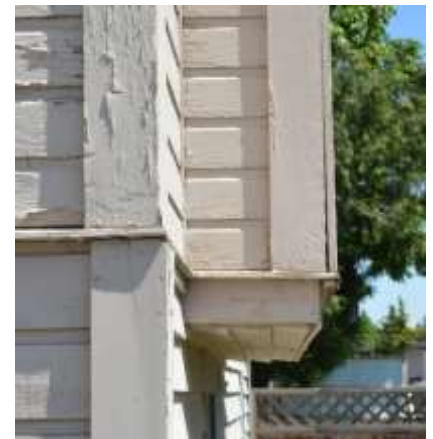
Figure 37: Corner boards at southwest corner
