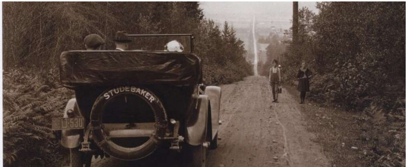
Figure 96: 1920: It shows a car on Pacific Highway about where 26th Avenue crosses, looking north towards Cloverdale. Note that the car is driving on the left. BC did not change to driving on the right until January first 1922. Photo by Leonard Frank JMABC LF.40894
