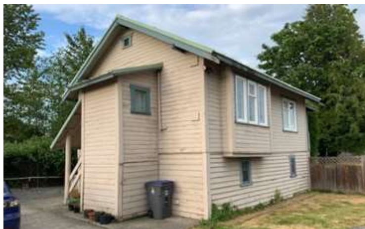
Figure 3: South-West corner (owner's photo)
