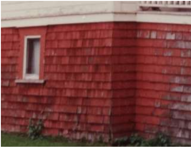
Figure 80: Straight mitered cedar shingles corner
