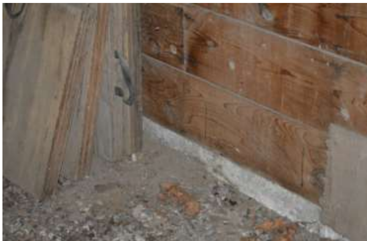
Figure 13: Extent of foundation beneath porch deck
