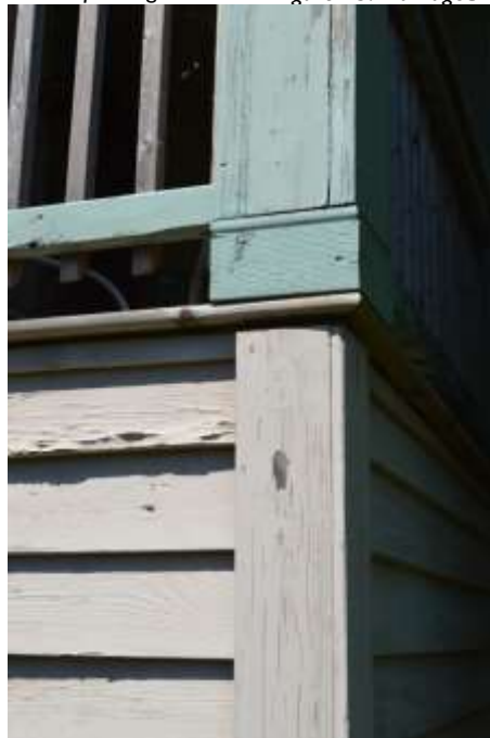
Figure 45: Lap siding below porch deck
