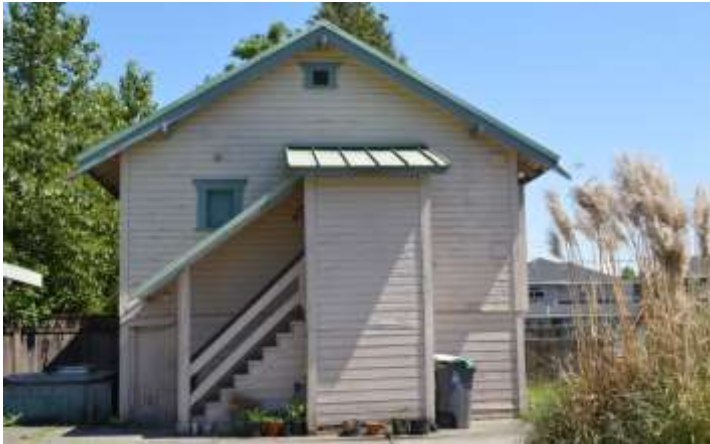
Figure 87: Back staircase with enclosed landing and storage below
