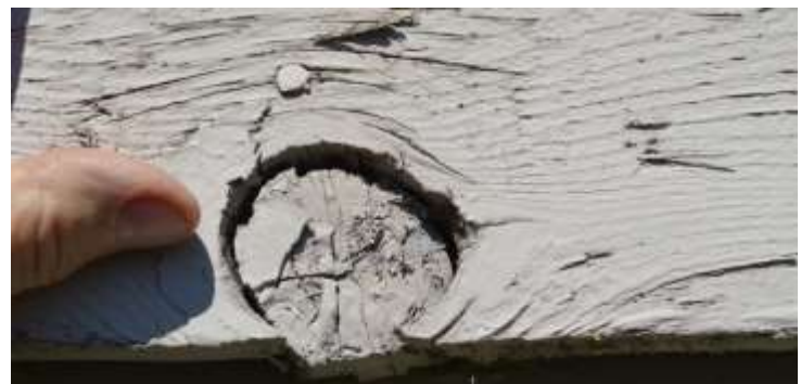
Figure 39: Rough wood siding boards with exposed knots
