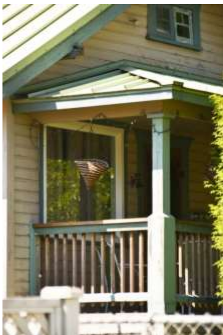
Figure 26: Standing seam metal roof at porch
