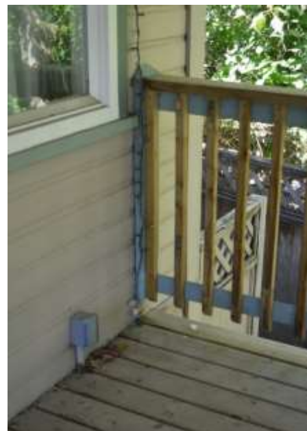
Figure 31: Balustrade at porch wall
