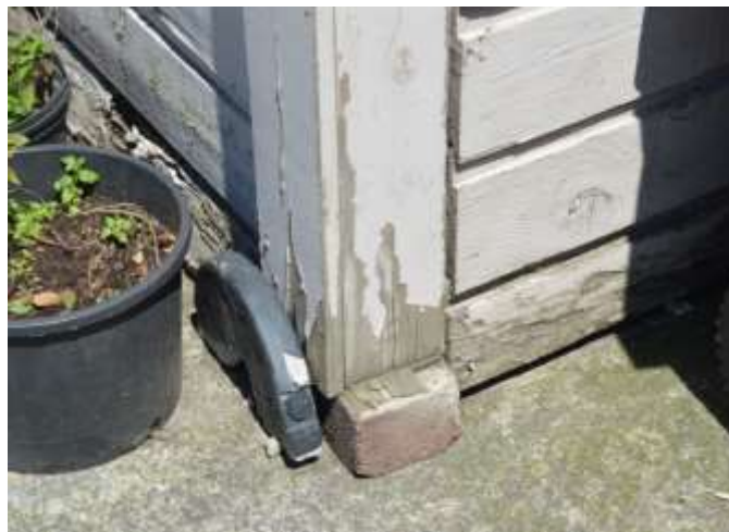
Figure 14: Brick supporting siding at south-west corner of back staircase
