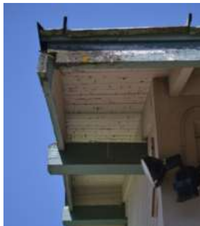
Figure 24: Open gable & exposed purlins
