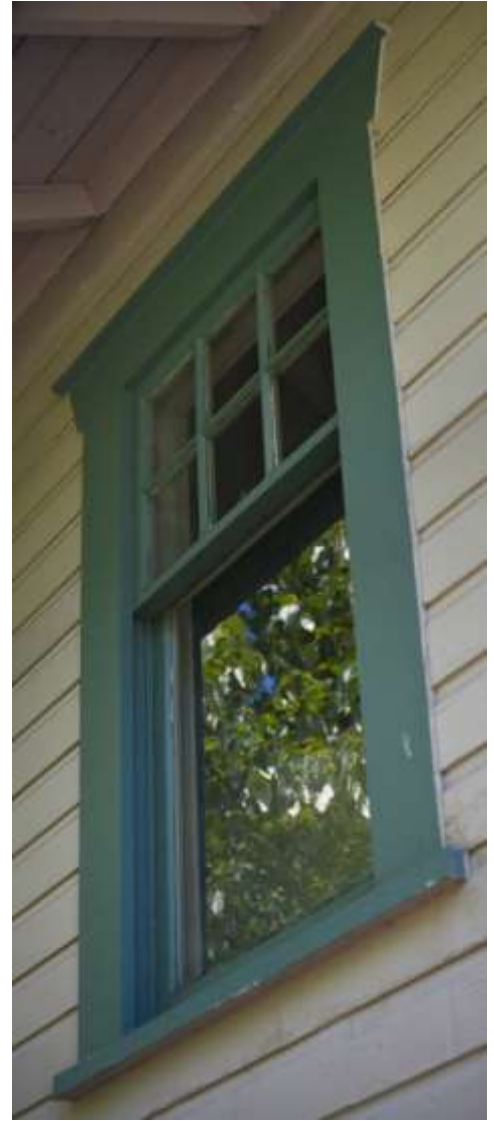
Figure 52: W07 Main floor north
