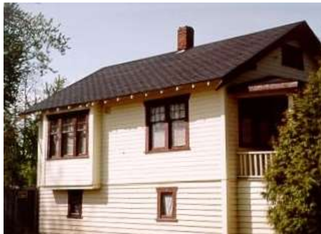
Figure 79: Asphalt shingles roof at the John Lamb House in 1998
