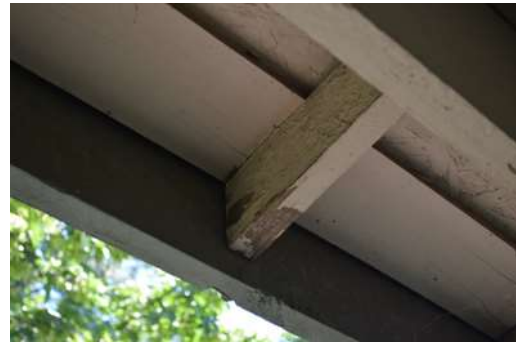
Figure 34: Detail of porch of roof overhang from below
