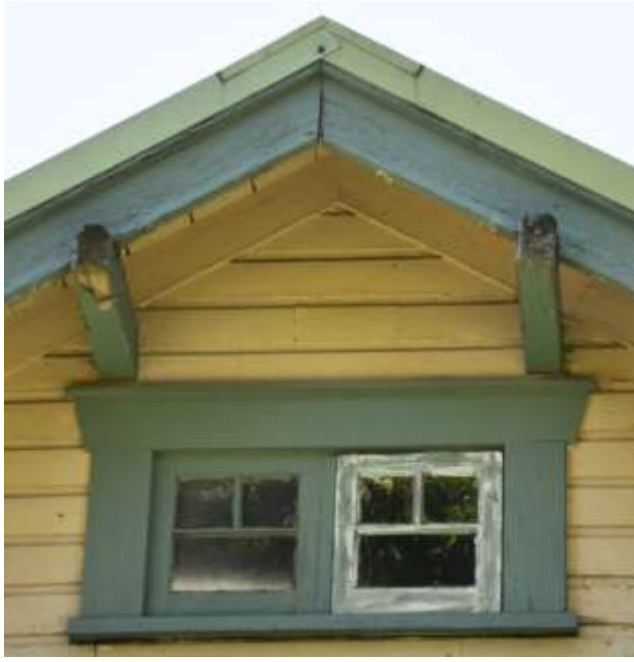
Figure 56: W13 Attic east, gable with purlin, headboard and barge board
