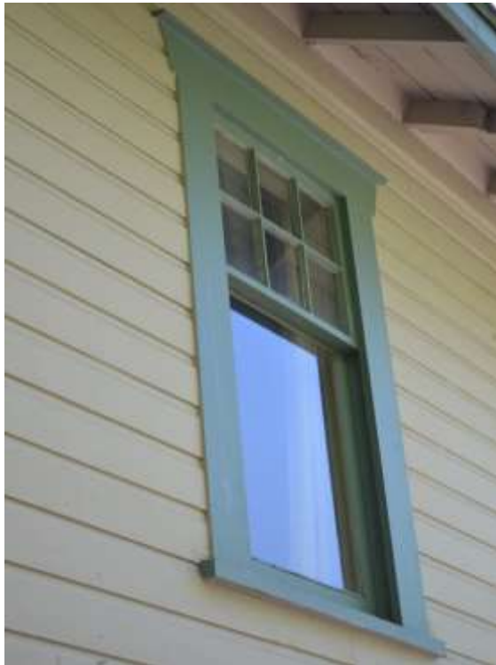
Figure 75: W07 Double hung window at main floor typical of the house
