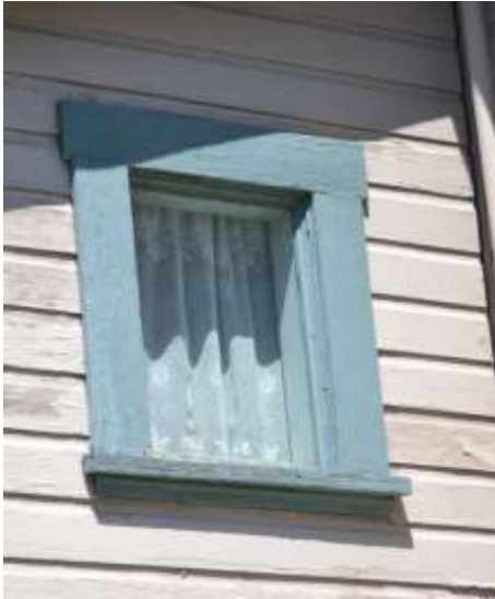
Figure 48: W05 Main floor staircase south wall
