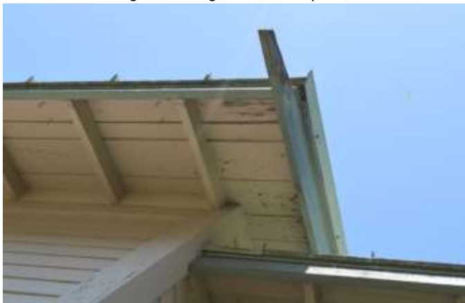
Figure 21: Open soffit, roof-underside and exposed rafters
