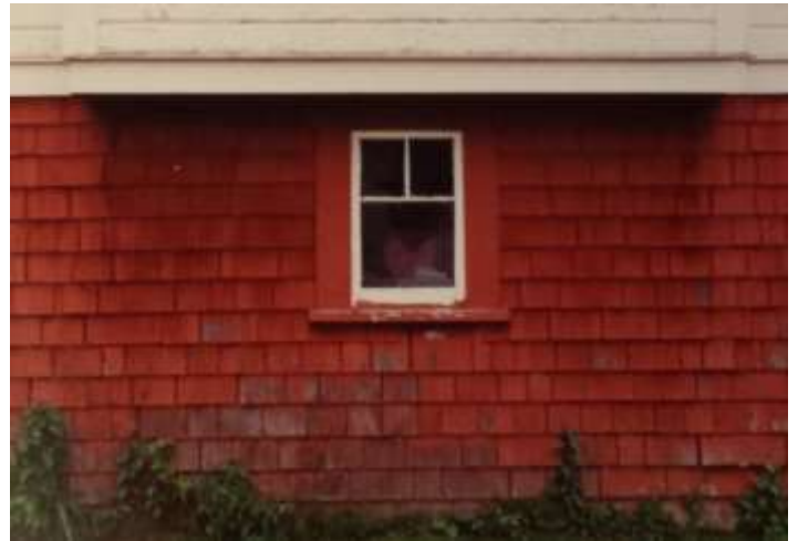
Figure 81: Ground floor shingle siding in the 1990's (Surrey Archives)
