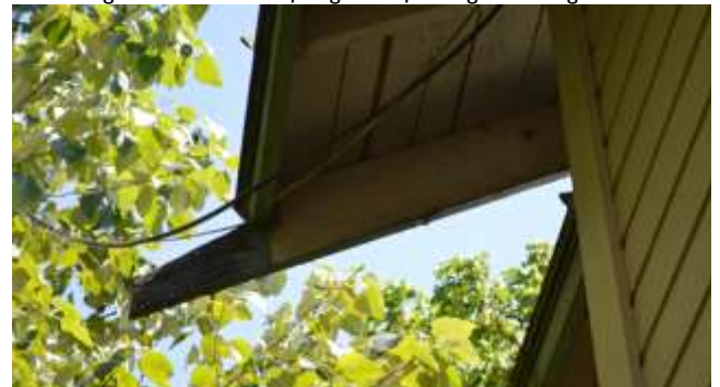
Figure 20: Barge board tapered tail
