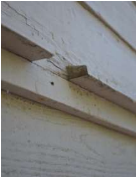
Figure 40: Belt moulding profile w/ base trim
