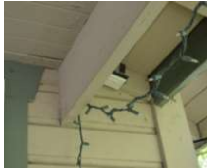
Figure 33: Porch framing beam at wall
