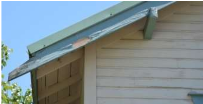
Figure 19: Barge board with tapered tail
