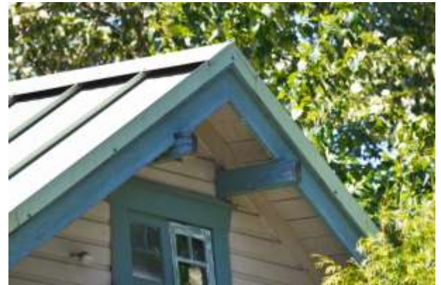
Figure 18: Metal roof ridge and flashing over barge board
