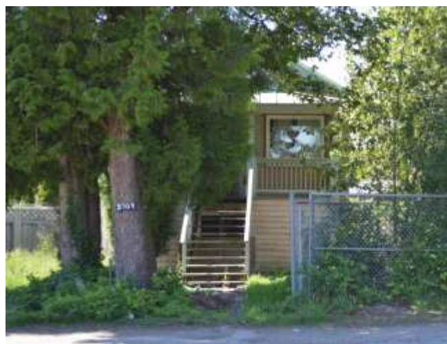
Figure 2: Front Porch facing 168 th Street
