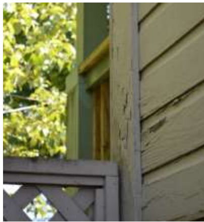
Figure 36: Corner board at northeast corner
