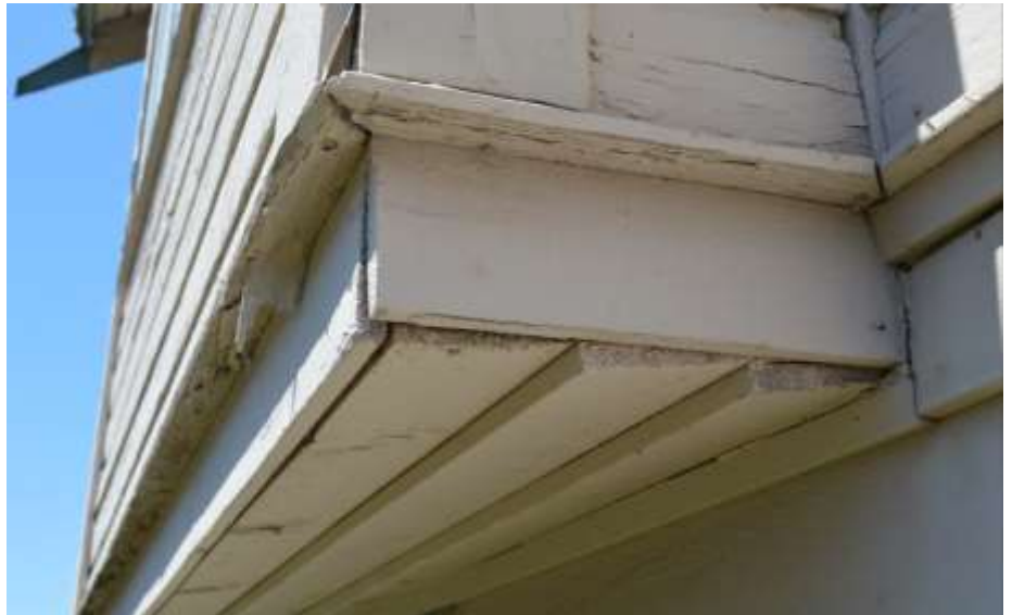
Figure 41: Belt moulding with base trim on the right and without at south face projection
