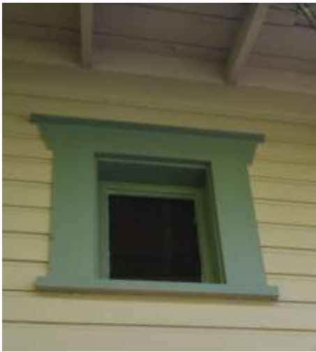
Figure 49: W08 Main floor north
