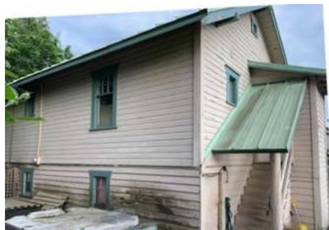
Figure 4: North-West corner (owner's photo)
