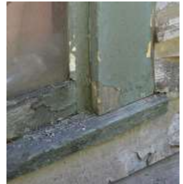
Figure 66: Sill, rail, stile and jamb
