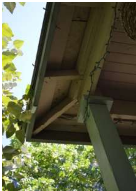
Figure 29: Porch post and open soffit corner
