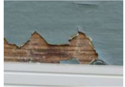
Figure 94: Window frame paint sample
