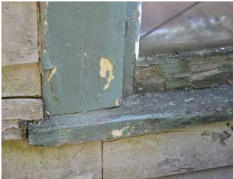
Figure 64: WII Sill, rail, stile and jamb
