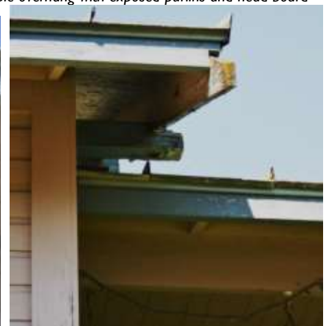
Figure 25: Southeast overhang and porch roof
