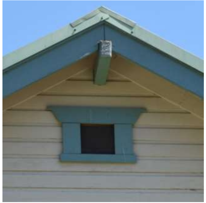
Figure 57: W14 attic west, gable with purlin, head board and barge board
