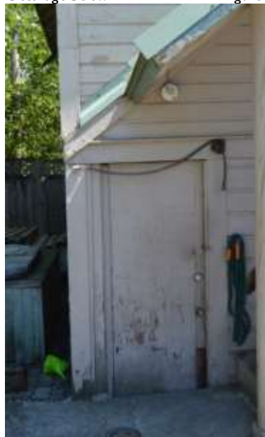
Figure 90: Storage door below stair landing
