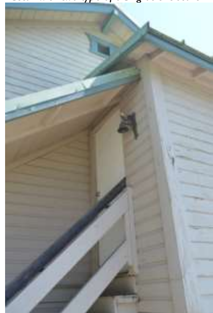
Figure 91: Door at top landing
