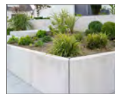
4. Concrete Retaining Wall
