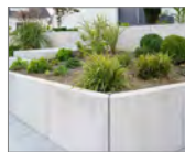
4. Concrete Retaining Wall
