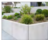
3. Concrete Retaining Wall
