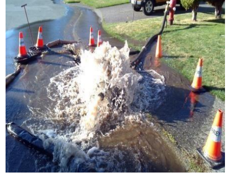
Typical set-up for water hydrant flushing
