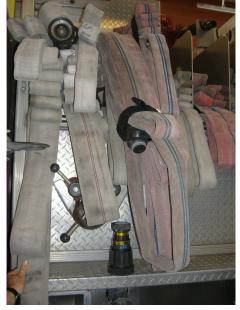
Figure 14 -- Surrey's pilot standpipe pack relies on 1.75 inch hoseline with combination nozzle. Removal of nozzle tip creates a smooth bore pattern.
