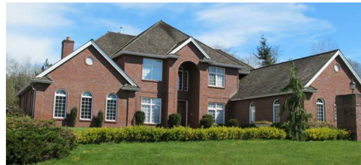
Existing Character-North Side of 26 Avenue (Photos taken at Orchard Grove)
