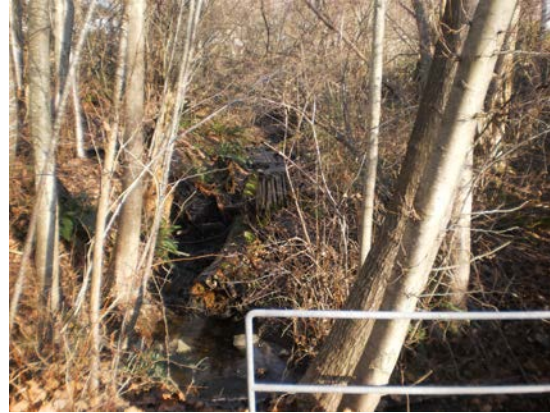
Photo: M. Creek near 84 th Ave. Signs of erosion
