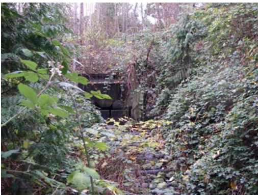
Photo: Hunt Creek outlet near 80 th Ave
