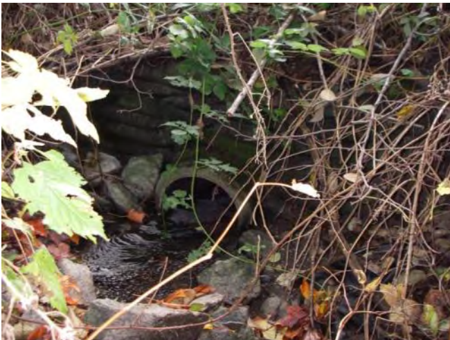
Photo 5. Hunt Brook headwaters, 300mm storm outfall originating near trailer park at 7850 King George.
