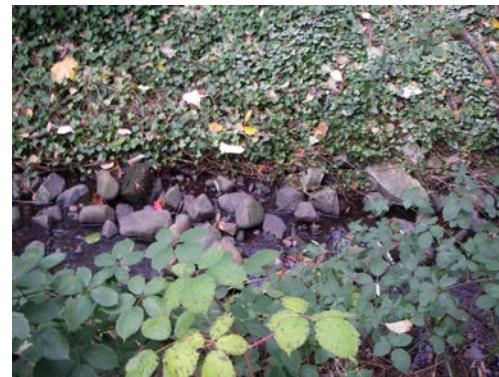
Photo: Erosion in Hunt Creek
