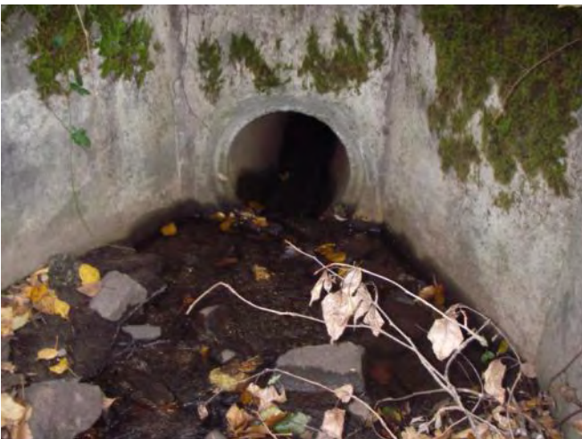
Photo 16. "M" Creek culvert at upstream end of 88th Ave.
