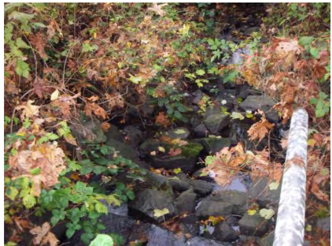
Photo 17. "M" Creek downstream conditions of 88th Ave culvert.
