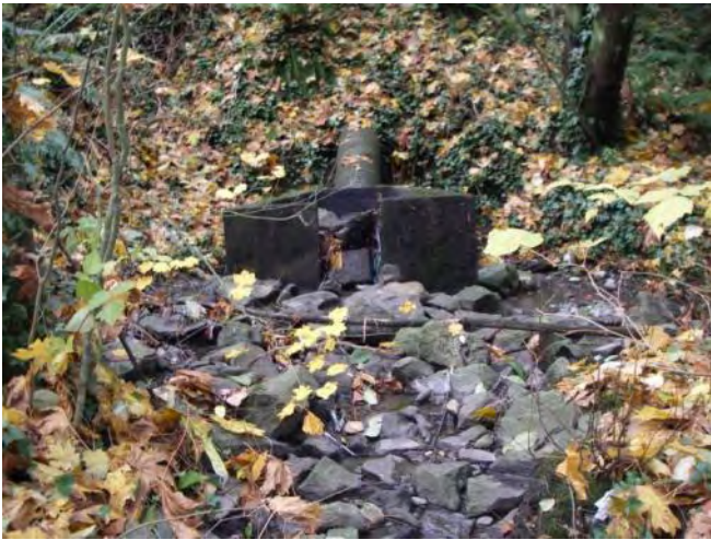
Photo 3. Hunt Creek headwaters, storm outfall.
