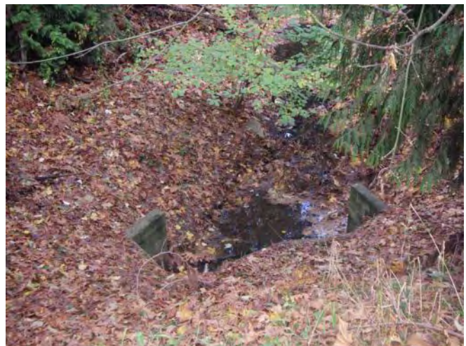
Photo 11. Beam Creek looking downstream from 78A Ave culvert outfall.
