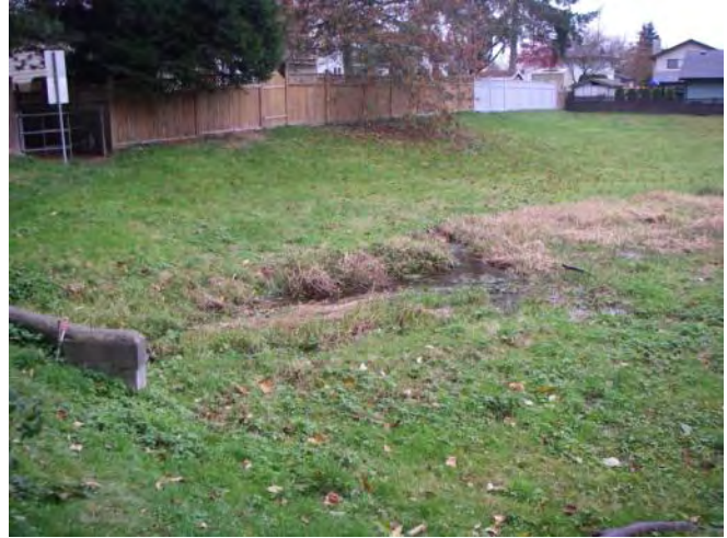
Photo 19. Enver Creek tributary culvert discharge near 92nd Ave.
