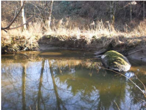
Photo: Bear Creek Erosion at 144 th Street
