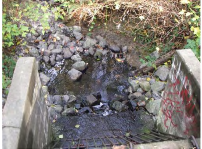
Photo 2. Outfall near 76A Ave. with recently placed rip rap.
