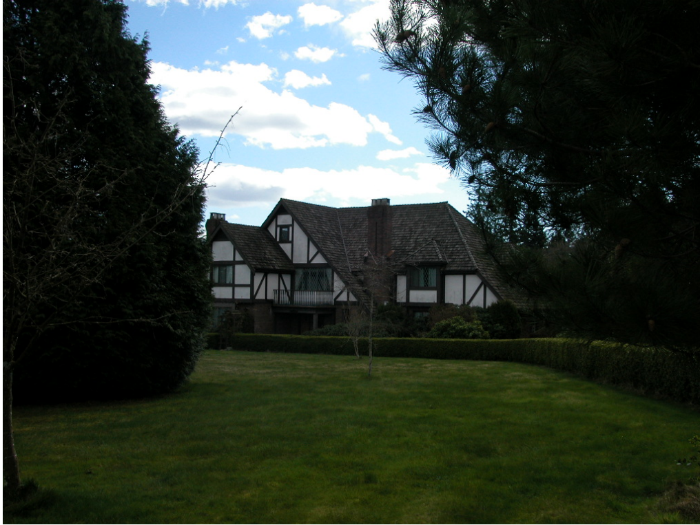
Tudor Revival house, NCP 2 (Photo: Hal Kalman)
