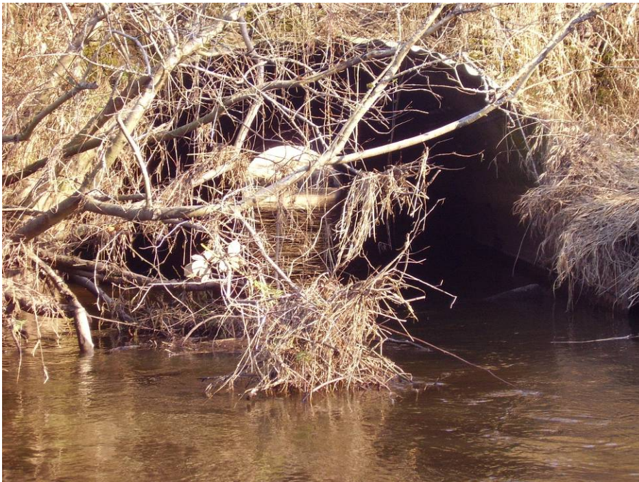
FIGURE 6-21 Photo of the Highway 99 Culvert Inlet
