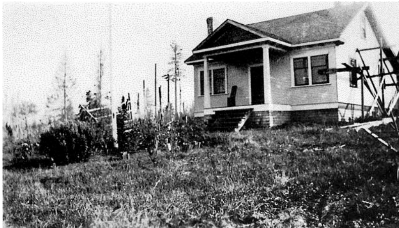
Figure 18: The house built by Charlie Perkins in 1927 on the southeast corner of Townline Road (96 Avenue) and Halls Prairie Road (184 Street), where he and his wife Nellie and family lived until his death in 1986. The "Big Tree" can be seen in the distance just to the left of the house and became a "hot topic" during the building of the #1 Highway. (courtesy Larry Perkins)
