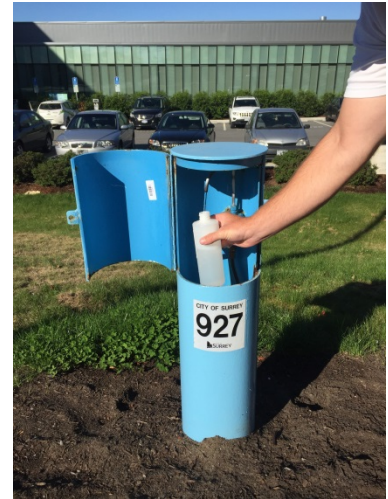
Water Sampling Station at 148 ST and 66 AVE
