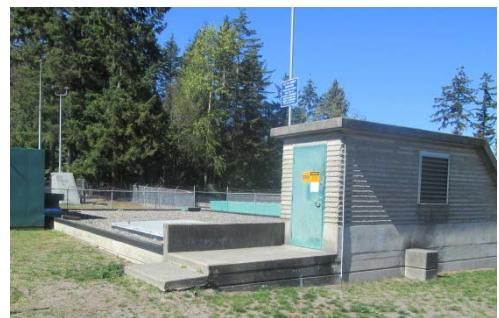
Newton Pump Station Sept 13, 2016
