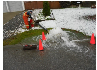
Typical set-up for water hydrant flushing.
