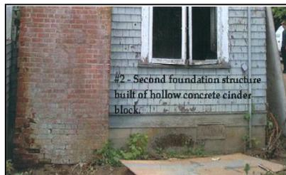
Prior to the 1900s houses generally were not built on concrete foundations so it was likely that the original farmhouse was built on a wood foundation and the basement was later dug out and the foundation installed. This West block or section was made larger at some point in time as evidenced by the concrete block foundation that it now rests on outside of the original foundation.
