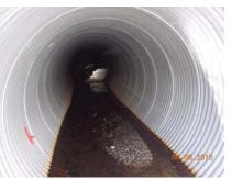
Photo 32. Looking in culvert shown in previous photo. Note side baffle plates and gravel.
