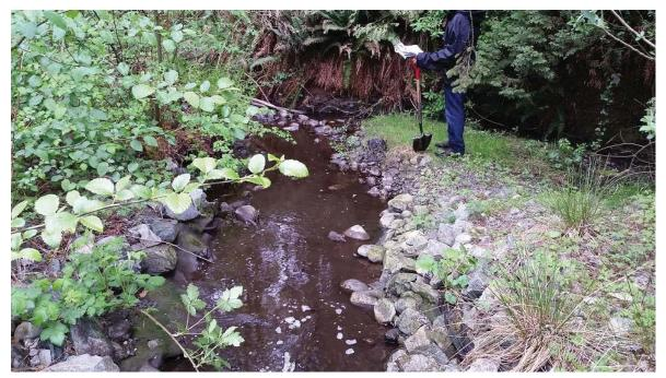
Photo 2. (WP20-1) Leoran Brook (upper section at Hwy 1). View of right bank erosion and recent instream works (~5 yrs old).
