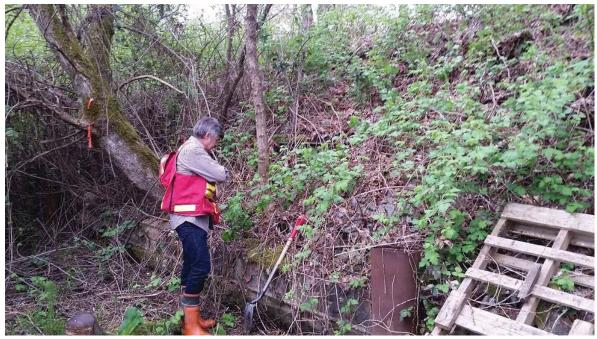
Photo 17. (WP18-SOLDIER PILES). Lyncean Creek West. View of left bank tiered solderpile walls (~300mm steel pipe piles with various metal lagging).
