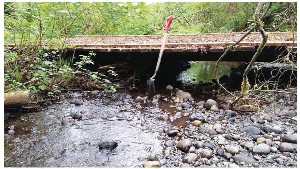
Photo 5. (WP20-BRIDGE). Leoran Brook (middle section). View of amatuer footbridge crossing with woody debris accumulating under the bridge against the stringers.
