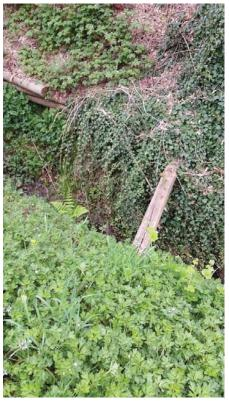
Photo 1. (WP-182A ST DITCH) 182A Street Ditch. View of left bank decaying and toppling landscape tie retaining walls and wall debris.
