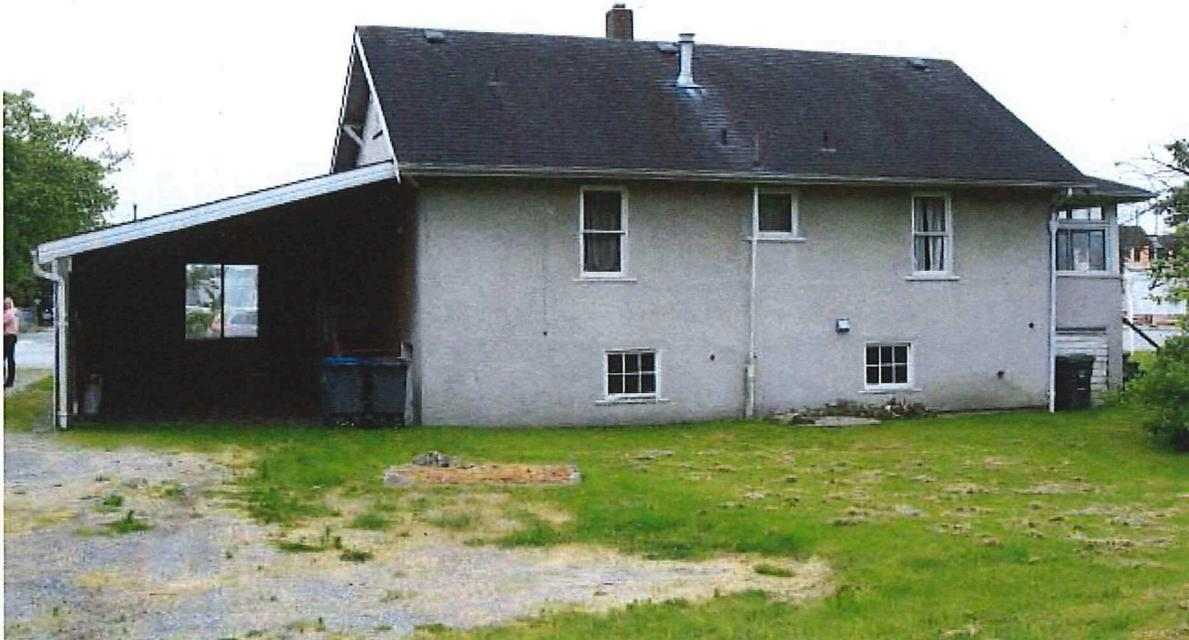
*Side (north) elevation of Main Residence, showing later shed-roof extension to the rear (left) and front verandah (right). Note uniform settlement at northwest corner of front verandah.*
