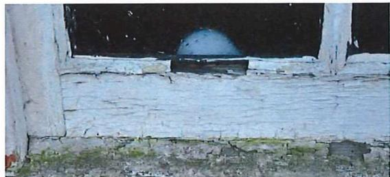
Photo showing typical deterioration of existing wood sashes.
