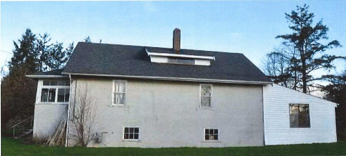
South elevation showing primary front-gabled wood-frame roof structure, shed dormer, interior brick chimney, hipped-roof (verandah), and shed-roof (rear extension, not original).
