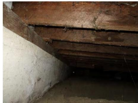
The floor structure is capable of meeting the assembly loads in compliance with the current building code.
