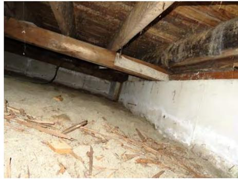
The floor joists are rough cut 2x8 spaced 18" running parallel to the shorter walls, about 20 feet in length. The floor joist are seated on the perimeter foundation beam and on the centrally located 6x6 rough cut beam so that the active load bearing length of the joists is 10 feet. The beam is supported by piers consisting of a combination of concrete blocks, 6x6 timber and 2x8 RC lumber. The joists are shimmed by lumber wedges where required. The floor boards appear to be 2x8 RC lumber.
