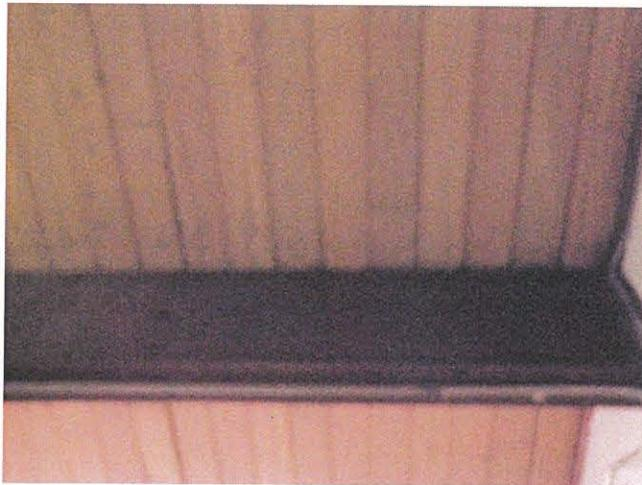
2x6 T&G ceiling over 5x17 glulams roof structure over the garage addition. The Glulams are not connected to the posts and the posts are not anchored to the concrete footings.
