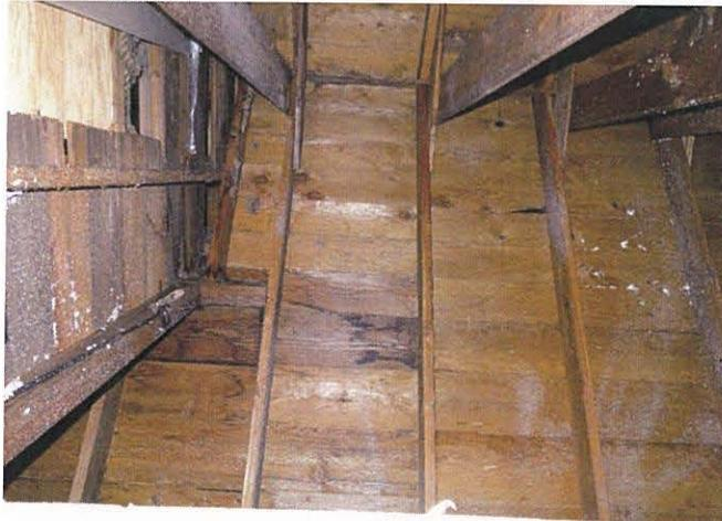
2x4 rafters @ 16" o.c. with 1x6 ridge beam and ridge collar tie with 1x6 crown post; twinned 2x6 queen struts connected to 2x6 @ 16" ceiling joists acting as tie beams.
