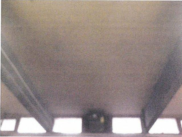
At the east wall of the garage addition the glulams are inserted into a steel framed window structure that is connected to the top of the bearing wall.
