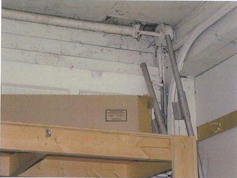
Original 3x2x12 beam inside the workshop wall in the ground floor; the beam is not connected to the 6x6 posts.
