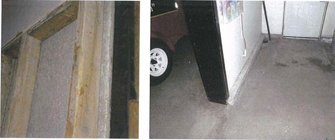
Opened west bearing wall of the addition attached to the original east exterior wall of 2x4 @ 16" framing on concrete strip footing. The wall is not anchored to the concrete footing.
