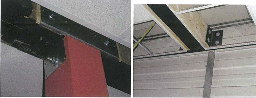
The two ceiling beams are unevenly loaded and the easterly one was strengthened in 2014 in recognition of the additional roof load transferred onto it by second story interior bearing wall. Also lateral movement was fixed by adding proper connectors at interface with posts and at end seats (see photo below).
