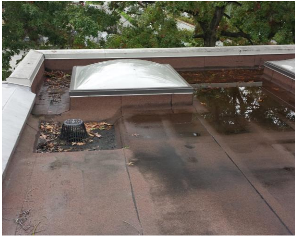
Figure 4: Ponded water observed on the roof at the south side of the stairwell
