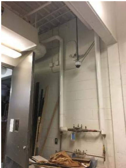
Figure 3 – Existing DCW main connection for Humidifiers
