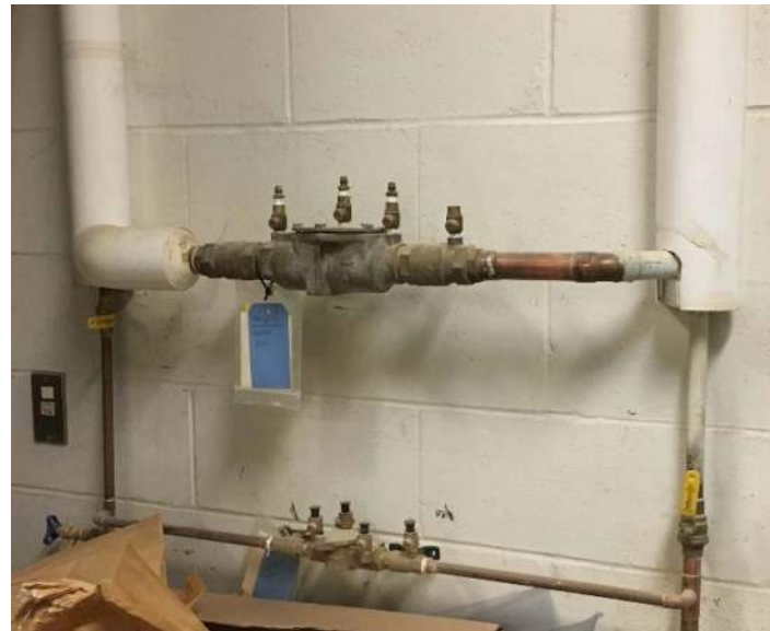
Figure 4 – Existing backflow preventer
