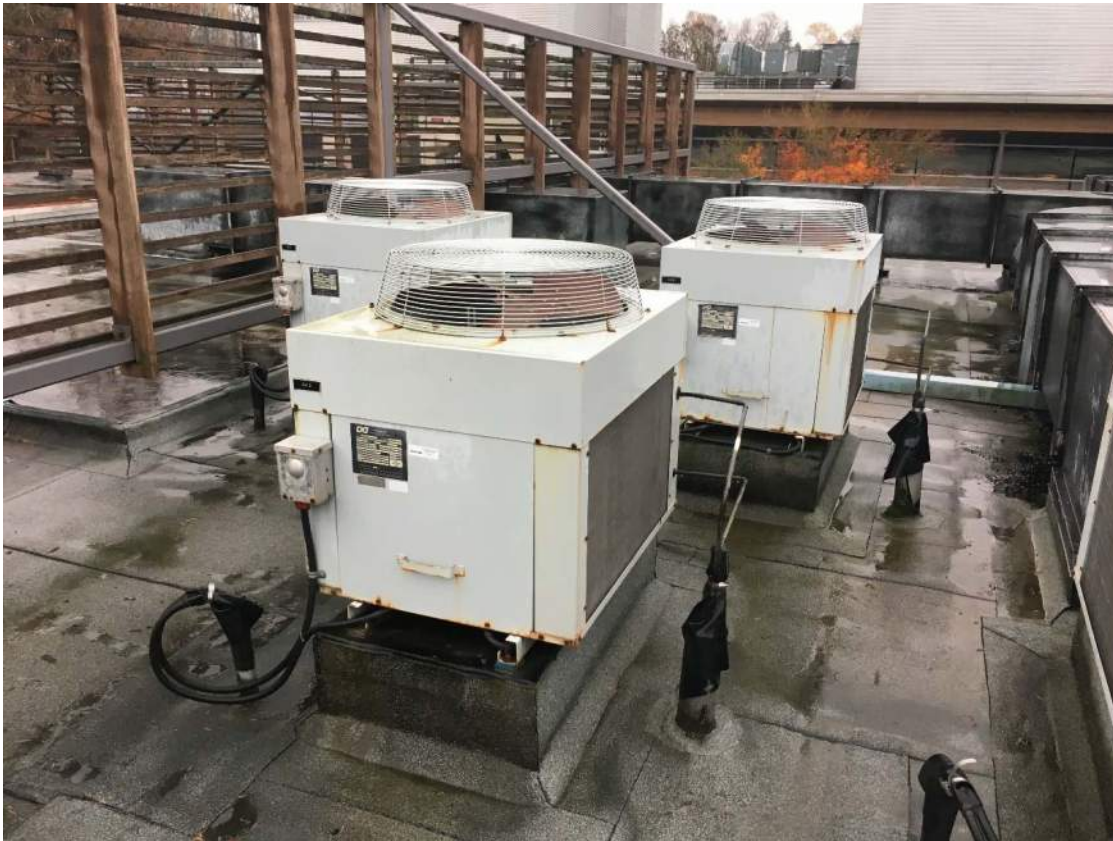
Figure 2 – Existing Condensing Units /w roof curbs & refrigerant piping roof penetrations (typical)
