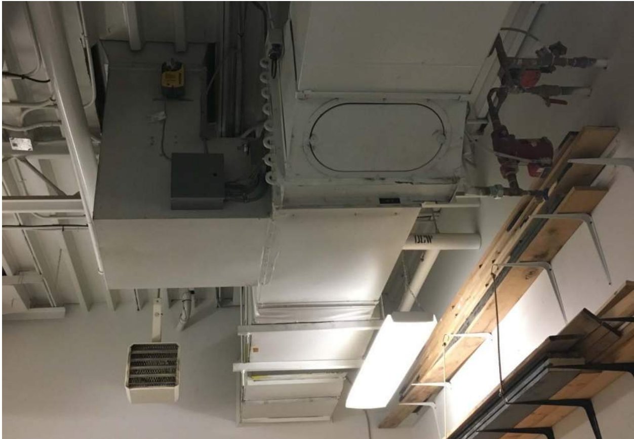
Figure 1 – Existing HWS/R lines for connection service to AHU-7
