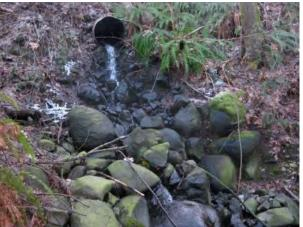
Photo 26. Unstable Boulders – Shadow Creek culvert outlet at Queen's Place.
