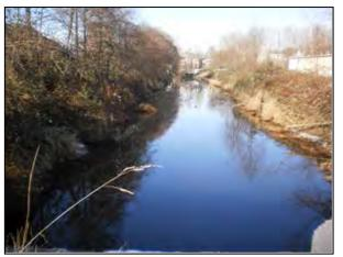
Manson Canal at Timberland Rd. 13m width, 2.4m height, 2H:1V Side Slopes.
