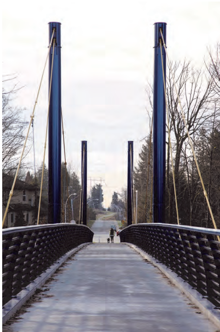
North Creek Bridge
