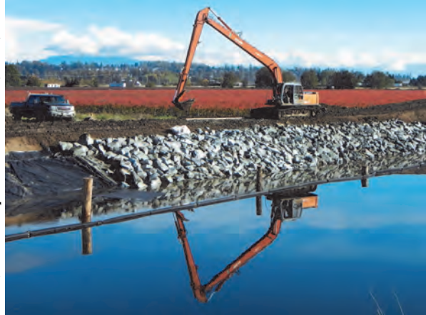
Burrows Pump Station erosion repair
