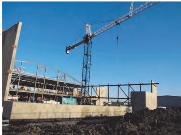
Cloverdale Recreation Centre
