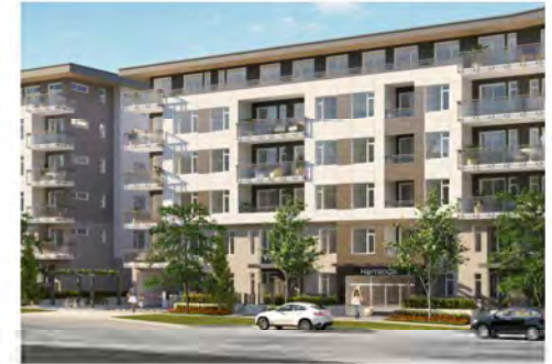
Two storey townhomes units will front King George Blvd. to differentiate the mixed use and residential buildings.
