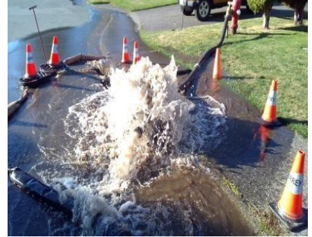
Typical set-up for water hydrant flushing
