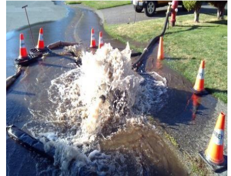
Typical set-up for water hydrant flushing
