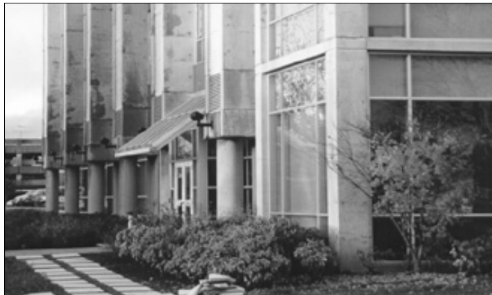
Landscaped setbacks and unit pavers maximize infiltration and define the building entry. The glass awning provides weather protection and allows light into the foyer.
