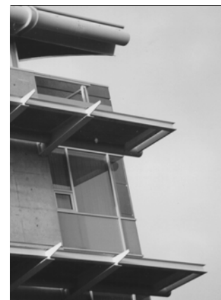
Light shelves provide shade to south facing offices and animate the facade.
