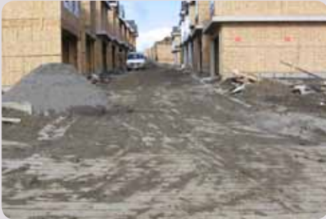
The above demonstrates inappropriate stockpile handling, and dirt accumulated on the road from construction sites with no BMP's. The accumulated dirt is then tracked further by site traffic.
