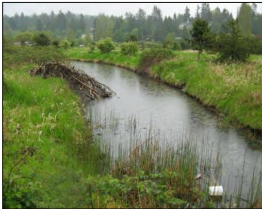
Dunsmuir Channel at Dunsmuir Road / Gilley Street intersection (looking east)
