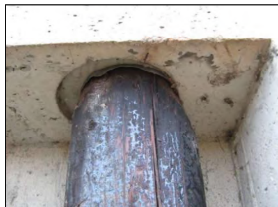
Timber pile and cap
