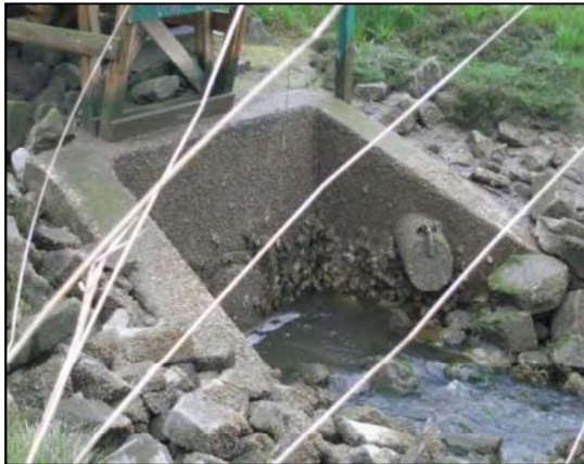
Flood box and pump station discharge pipe outlets
