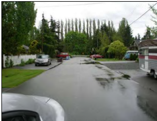
Ill defined drainage paths on local roadways
