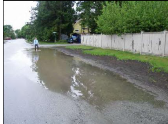
Surface ponding near McBride Ave and Target St following a rainfall event in May 2008
