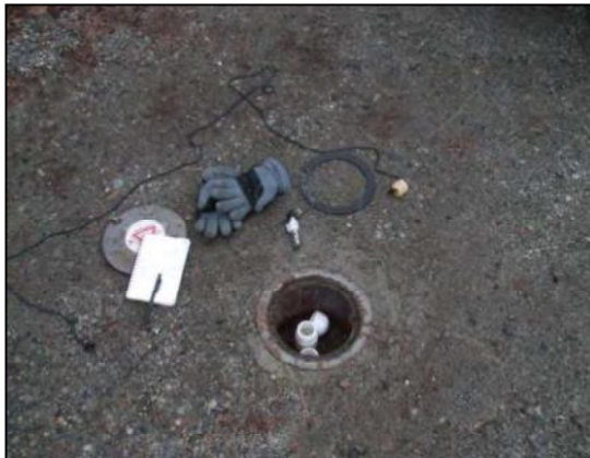
Groundwater monitoring well
