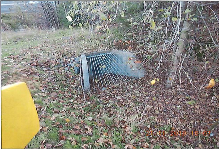
Photo 3: Culvert inlet at Hwy 10, no water present.
