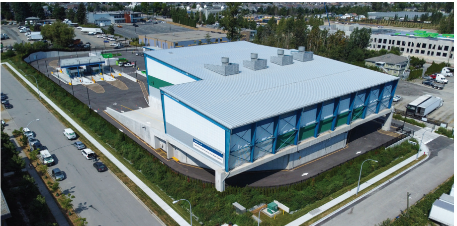
Central Surrey Recycling and Waste Centre
