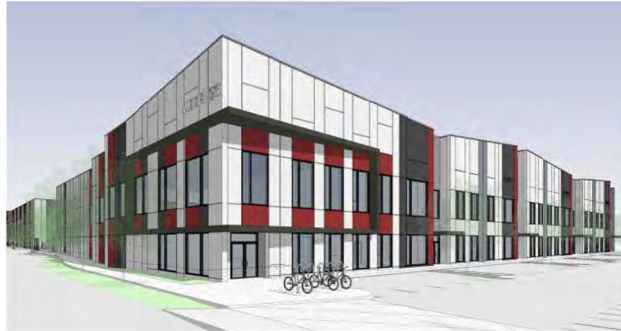
Building D from South West
