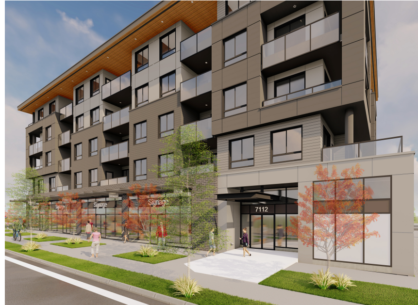
South West View from 128 street
