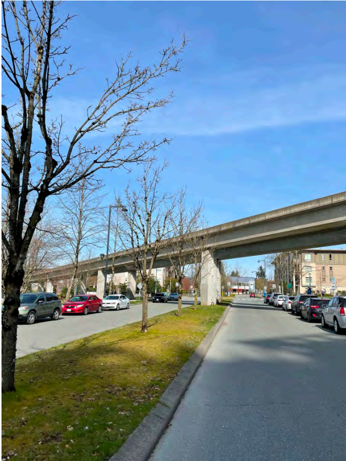
Figure 6. City trees within Gateway Drive median.
