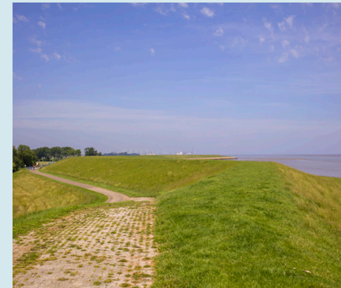
Raised dyke protects from storm surge and accommodates trails and other uses
