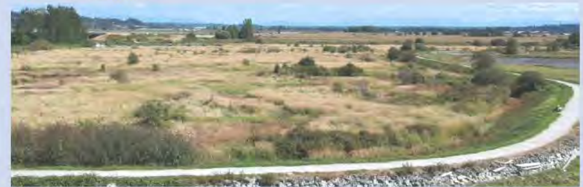
Maintain flood infrastructure: raised dykes
