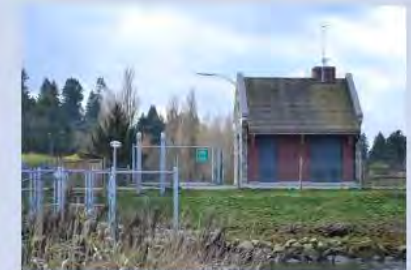
Maintain flood infrastructure: pump stations
