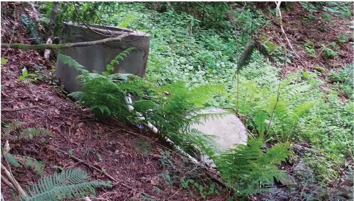
**Photo 12. (WP18-FILL/SUMP).** Lyncean Creek West (East Tributary). Small scale stormwater control structure (vandalized) flowing approximately 5gpm.
