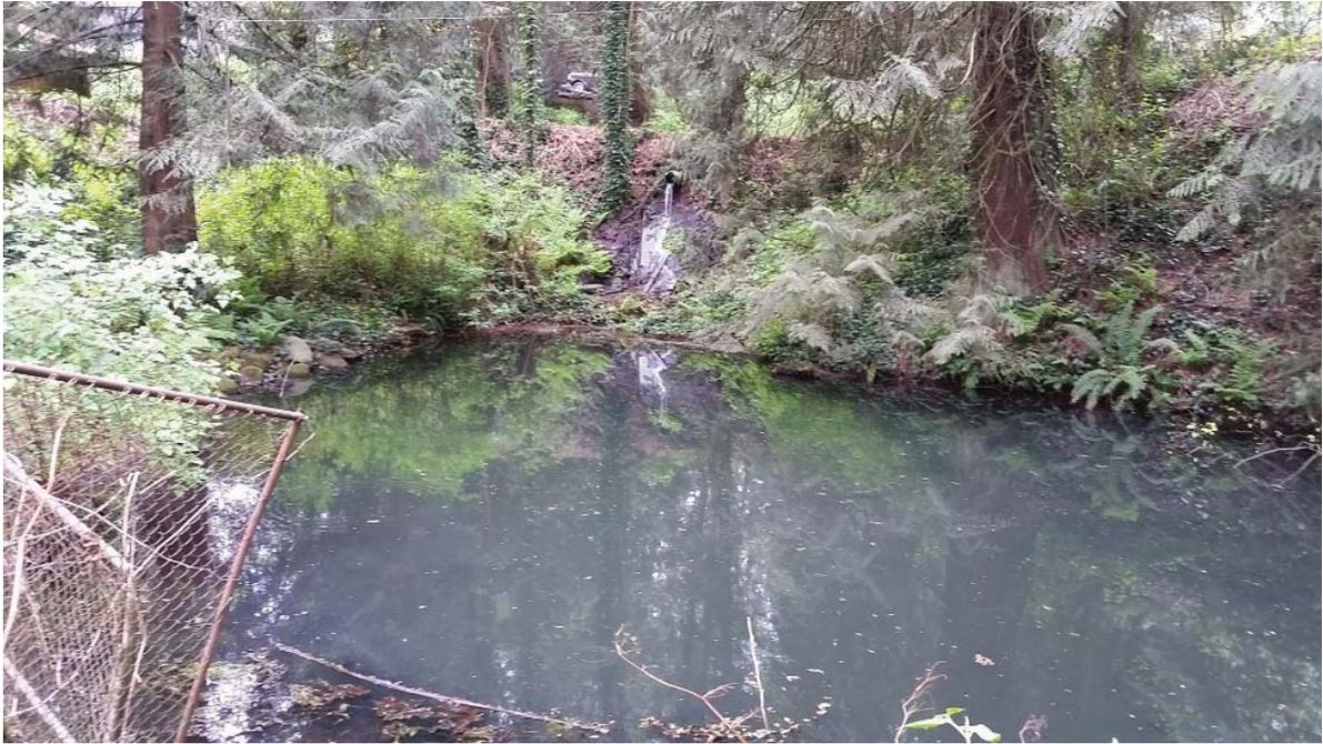
**Photo 9 (WP19-14).** Lyncean Creek East. View of main pond showing flow from upper pond through access road ravine fill. Main pond trash rack damaged and partially clogged with debris.
