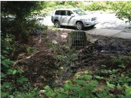
Photo 13. Artesian well outflow (enters storm culvert which discharges to Main Stream)
