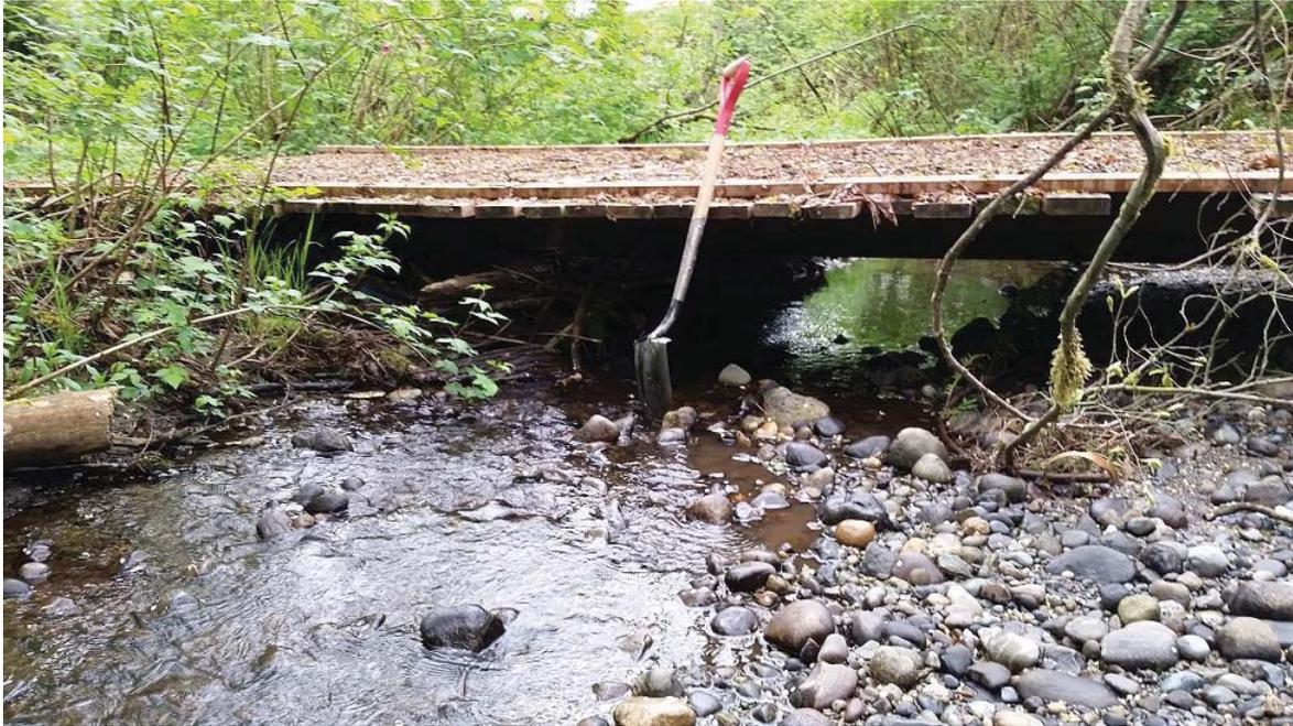
**Photo 5. (WP20-BRIDGE).** Leoran Brook (middle section). View of amateur footbridge crossing with woody debris accumulating under the bridge against the stringers.
