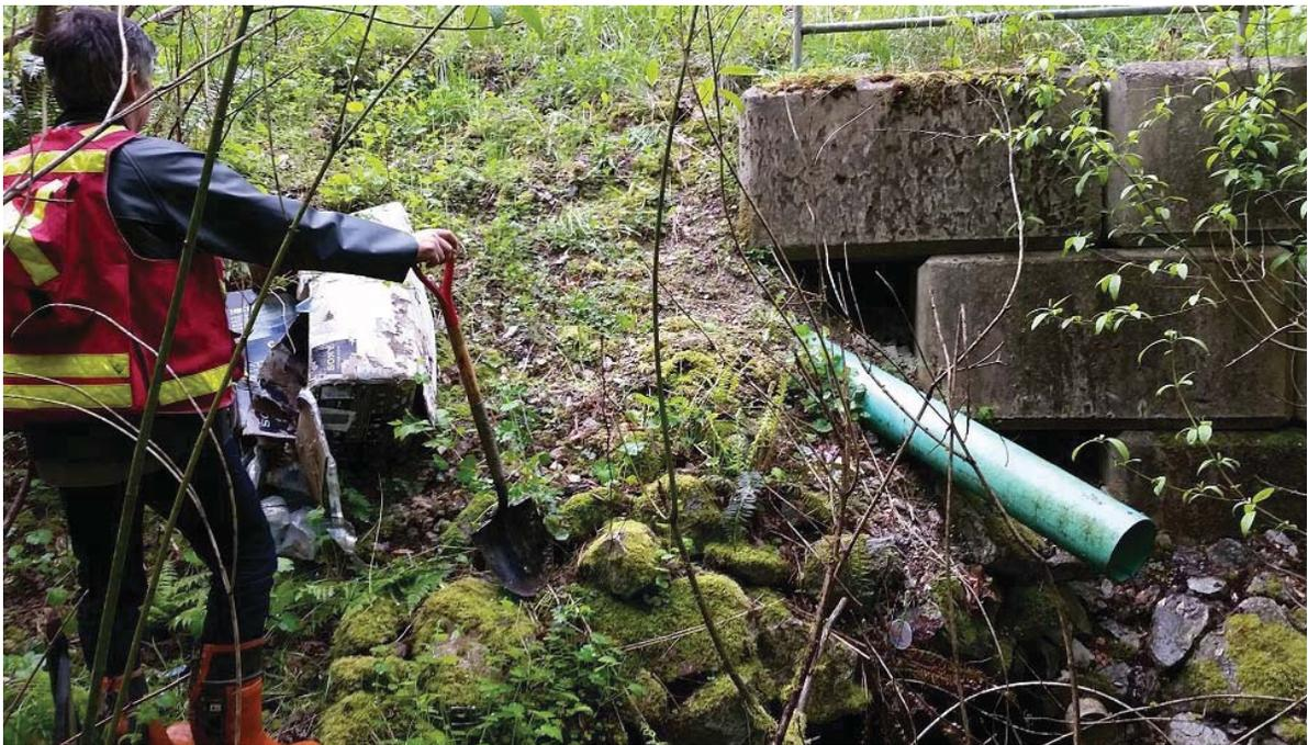
**Photo 10 (WP19-2).** Lyncean Creek East (179 Street culvert crossing). View of 200mm pipe draining northbound roadway scupper and Lock Block retaining wall erosion.
