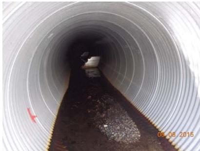
Photo 32. Looking in culvert shown in previous photo. Note side baffle plates and gravel.
