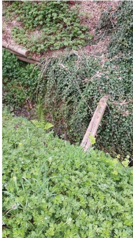
**Photo 1. (WP-182A ST DITCH)** 182A Street Ditch. View of left bank decaying and toppling landscape tie retaining walls and wall debris.
