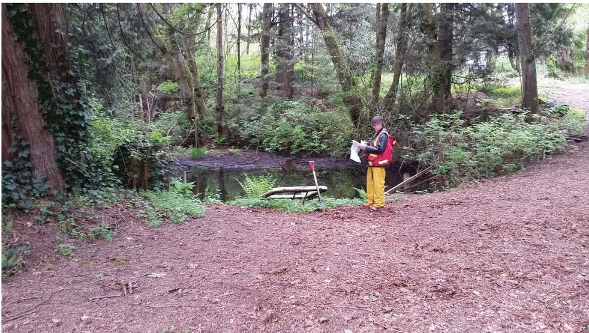
**Photo 8. (WP19-14).** Lyncean Creek East. View of upper pond (access road ravine fill). Culvert trash rack partially clogged with debris
