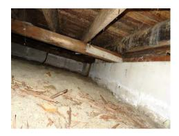
The floor joists are rough cut 2x8 spaced 18" running paralel to the shorter walls, about 20 feet in length. The floor joist are seated on the periemter foundation beam and on the centrally located 6x6 rough cut beam so that the active load bearting length of the joists is 10 feet. The beam is supported by piersc onsisting of a combination of concrete blocks, 6x6 timber and 2x8 RC lumber. The joists are shimmed by lumber vedges where required. The floor boards appear to be 2x8 RC lumber.
