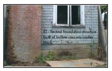
Prior to the 1900s houses generally were not built on concrete foundations so it was likely that the original farmhouse was built on a wood foundation and the basement was later dug out and the foundation installed. This West block or section was made larger at some point in time as evidenced by the concrete block foundation that it now rests on outside of the original foundation.
