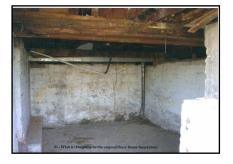
It appears that the first original farmhouse may have been smaller at one time than the current West block of the structure, as evidenced by the smaller foundation walls in the basement. They currently provide no structural support or influence on the building above.
