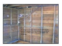
The gable ends also show the slope of the original roofline. At some point (probably before the Baron took ownership as the spacing of studs and rafters are 24 -30" apart) the owner extended the walls for a second storey and built a new roof complete with dormers.
